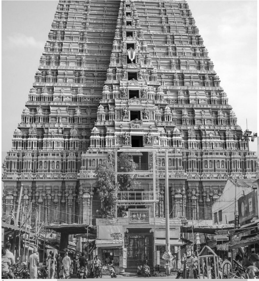
Twelfth tier completed – January 1984
