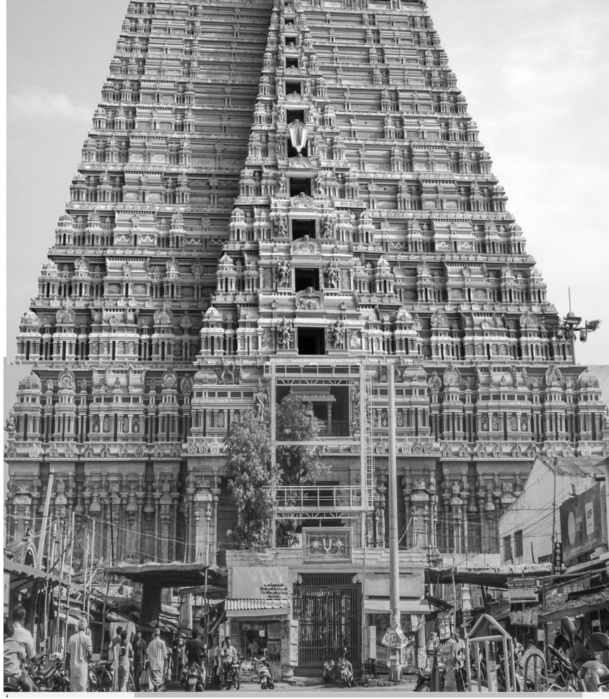
Thirteenth tier completed - April 1984
