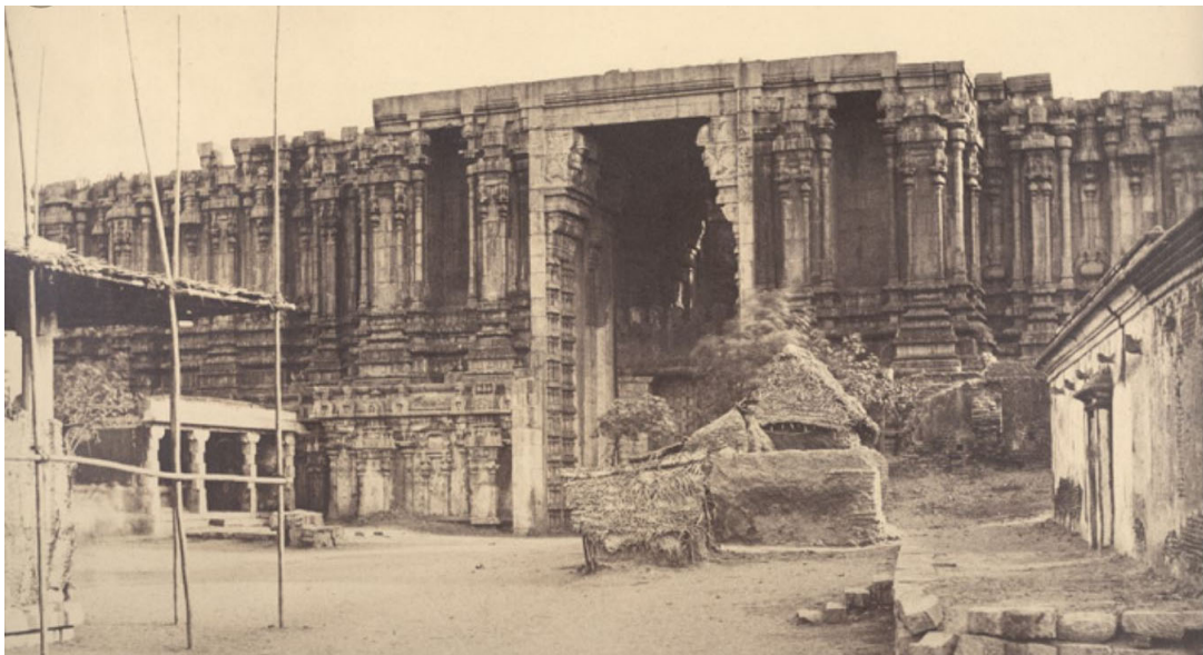
MoTTai gopuram – another view
