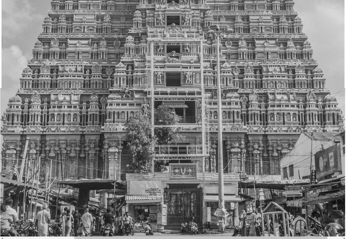
Fourth Tier constructed – July 1982
