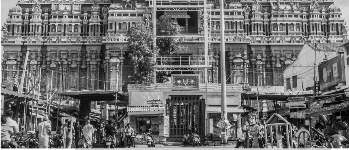
The First Floor constructed – October 1980
