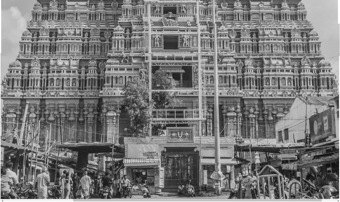
Third tier constructed – October 1981
