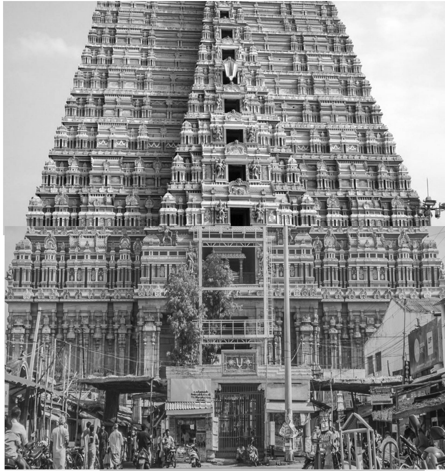
Tenth tier completed – December 1983
